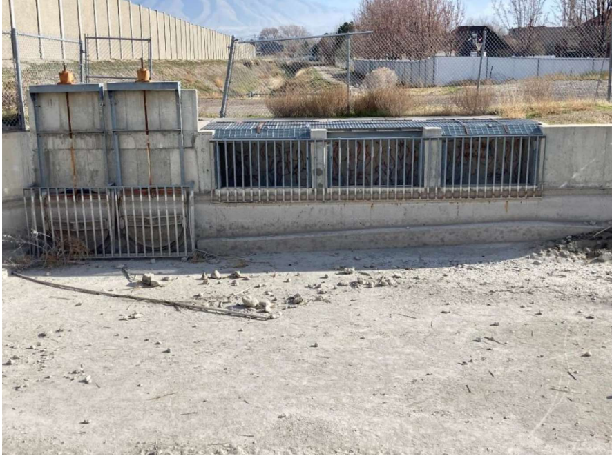
Photo 2-1: Overflow/Dump-Out Structure Where Utah Lake Distribution Canal Crosses Rose Creek
