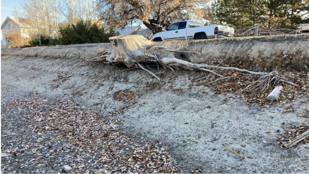
Photo 2-10: Tree Stump with Roots in the Utah and Salt Lake Canal Embankment
